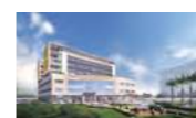
Establishing the UHS Teaching Hospital Project, Cambodia 캄보디아 UHS 대학병원 Design 2022, Completion 2027
